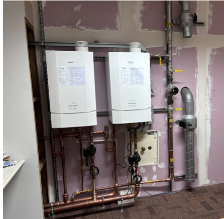
Work progressing with the new boilers in the Carrick Room
